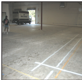
Before photo showing old concrete
