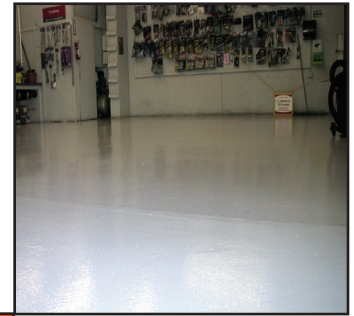
4800 over installation bay
