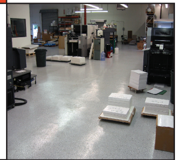
After photo, commercial printing plant
